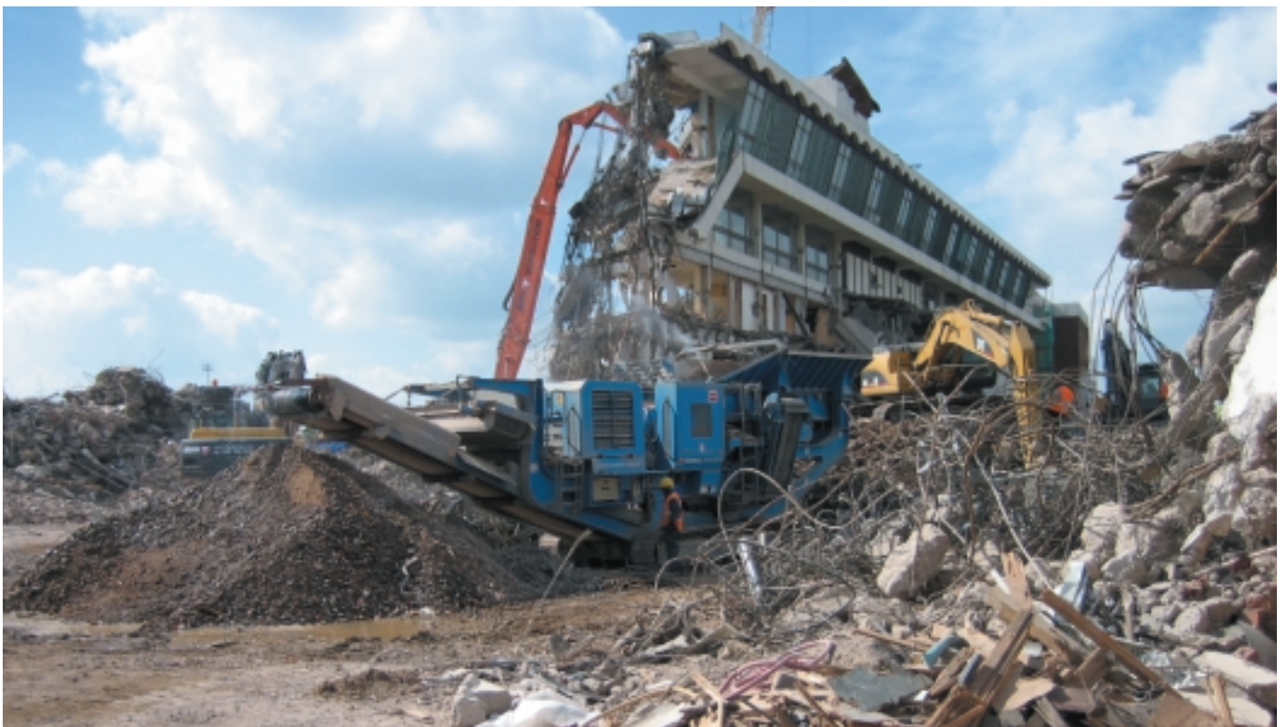
DONCASTER The demolition of the Yorkshire Stand commenced in spring 2006. The Board has approved a loan of £8m towards this major redevelopment project over the next two years.
