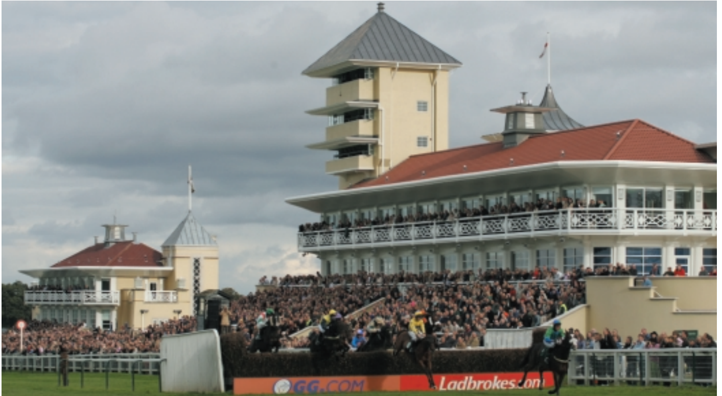
TOWCESTER The start of the 2005/06 season saw the opening of the new Empress Stand. Facilities include a new betting hall, and a restaurant and hospitality boxes on the first and second floors respectively. Officials also benefit from a new integrity tower.
